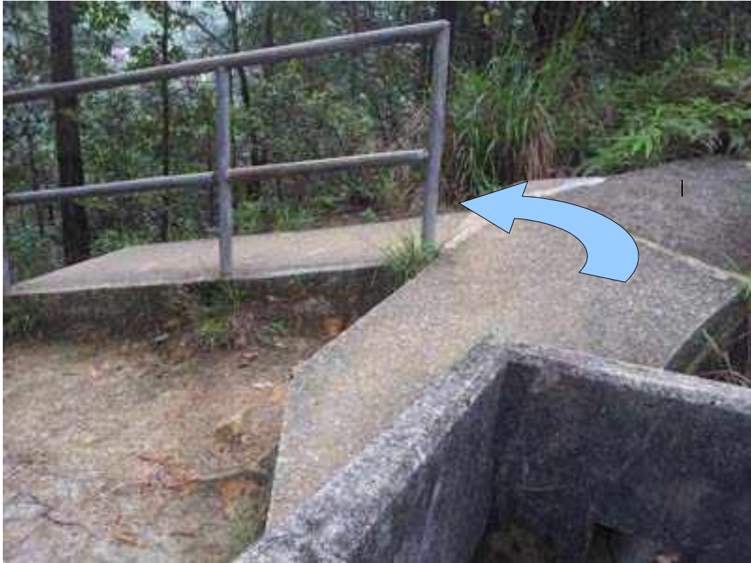
Left on cement path
