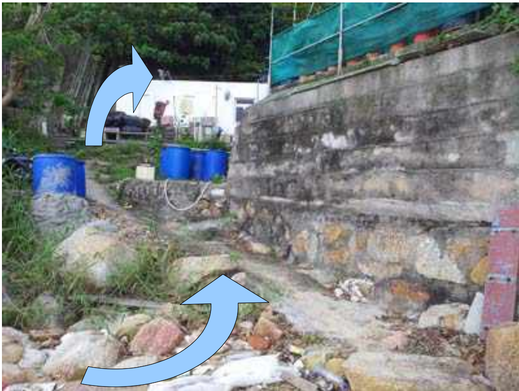
Left turn on beach – up short 10m trail to house and turn right on cement path to Nim Shue Wan
